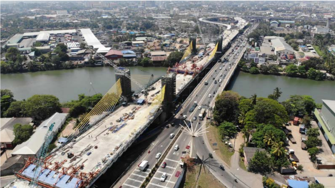
Image courtesy of Road Development Authority, 'New Kelani Bridge Project'
